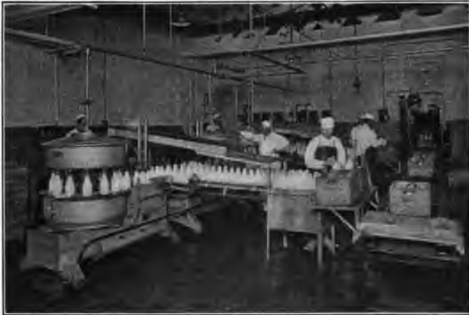
FIGURE 37. — INTERIOR OF MILK STATION.
